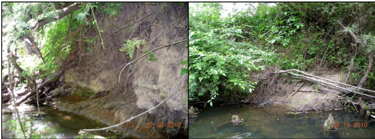
Ongoing channel incision and related active terrace bank instability and fine-textured sediment supply in (former) swampy-meadow reach of Butano Creek. Right photograph shows ancient trees (5-10 ka) which were recently exhumed by channel incision, within channel at base of valley fill.
