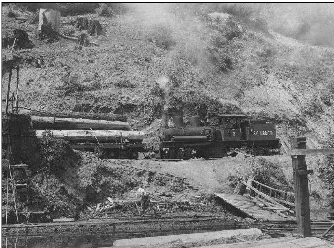
Santa Cruz Lumber Co. railroad along upper Pescadero Creek, in 1930s-1940s.
