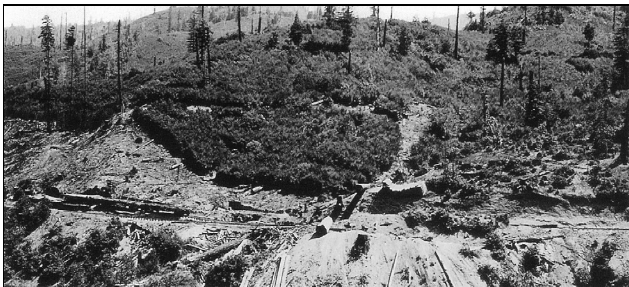
Santa Cruz Lumber Co. railroad along upper Pescadero Creek, in 1930s-1940s.
